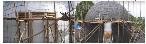
Fig. 6. Fixing of steel rebars and use of concrete.
