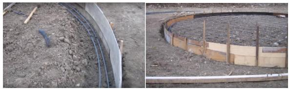
Fig. 4. Stages of construction showing the formation of base slab.
