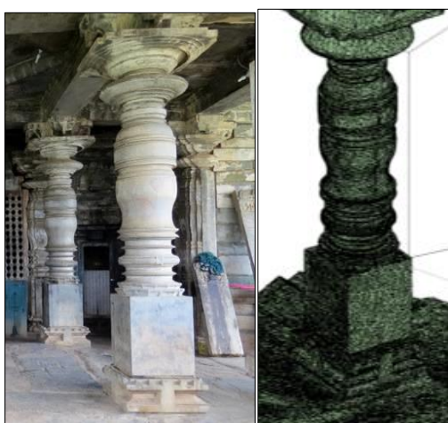
Fig. 2: Actual Photograph And A Screen Shot of 3D Scan Model of a Circular Column of Galgaganatha, A 11th century Temple of Haveri District.
